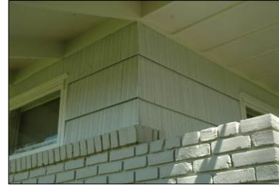
Use of multiple materials is a character-defining feature of some residences. Note the placement and patterns of the asbestos shingle and brick.
