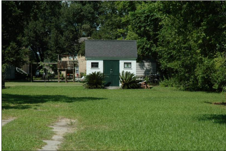
Example of a storage shed.
