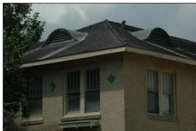
On this apartment building, the wide overhanging eaves, exposed rafter ends, and eyebrow dormers are important character-defining features.
