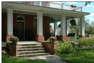
On this porch, the columns with brick bases and flat roof form with balustrade are character-defining features and should be preserved.
