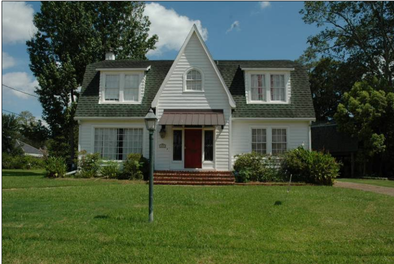
Local example of a Cape Code residence.
