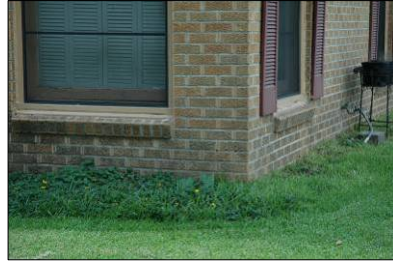
Note the textured brick and depth of the mortar joints in this exterior wall.
