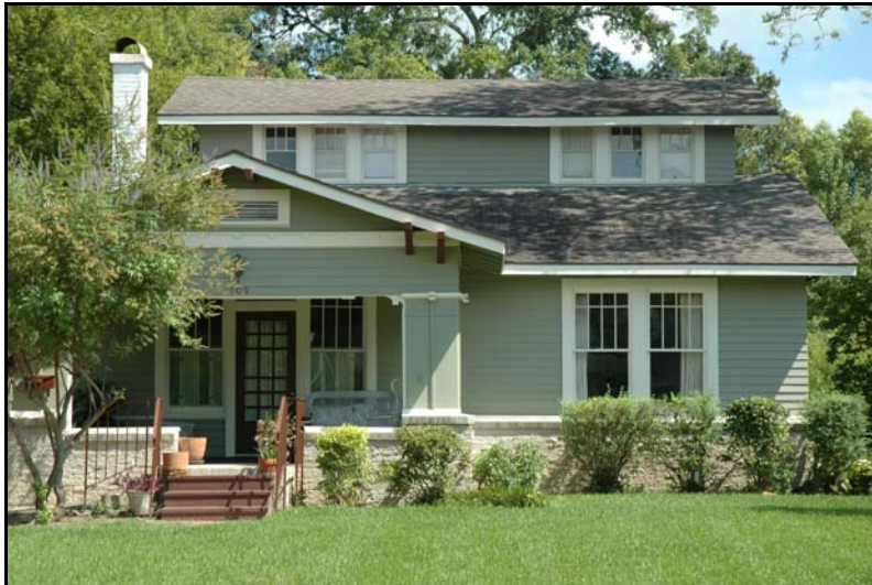
Example of Craftsman Style bungalow. Note brackets at wide overhanging roof eaves, tapered porch columns with wide bases, and multiple lights in upper sashes of windows.
