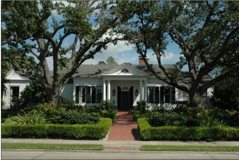
Example of a center passage residence.
