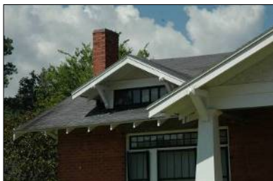
The dormer, with its shallow window and support brackets, is a character-defining feature of the roof of this Craftsman Style building.
