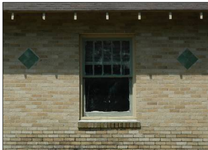
Note the five-over-one lite pattern of this double-hung wood-sash window.
