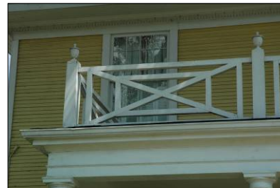
The fretwork balustrade on the roof of this Classical Revival Style house is an important feature that should be maintained.
