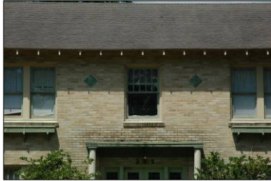
The character of an exterior wall is defined by its texture, color, and pattern. Note use of brick and terracotta tiles.
