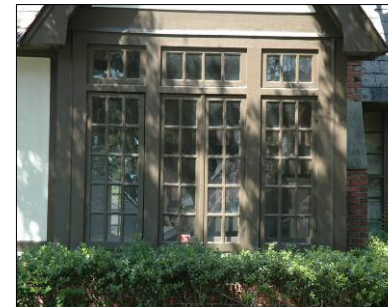
Operable wood casement windows complement this residence.
